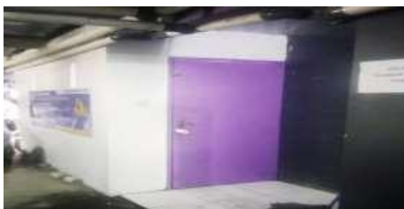
Fig 4. Generator room building
