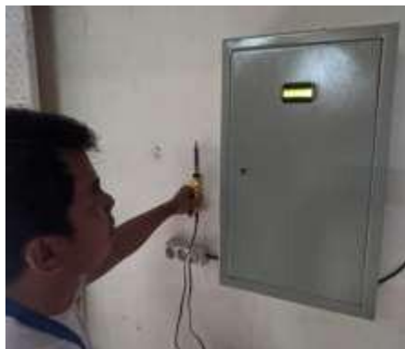
Figure 17. Solder Load Testing
